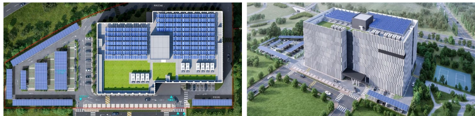
Dongtan Data Center Solar Power Generation Facilities
